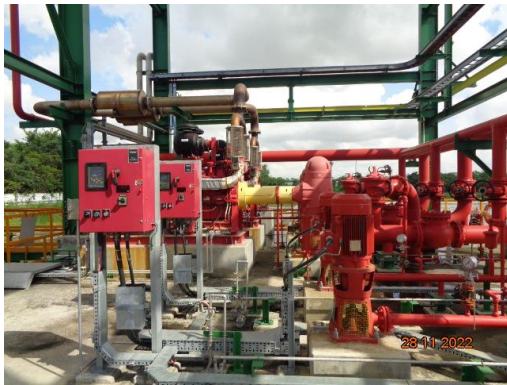
Electric Motor Driven Jockey Pumps
