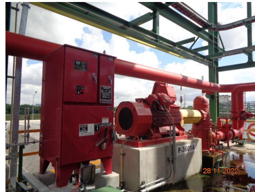
Electrical Driven Fire Water Pump
